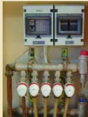
smartcontrols operate thermo-electric actuators at the distributed manifolds for an underfloor heating system.
