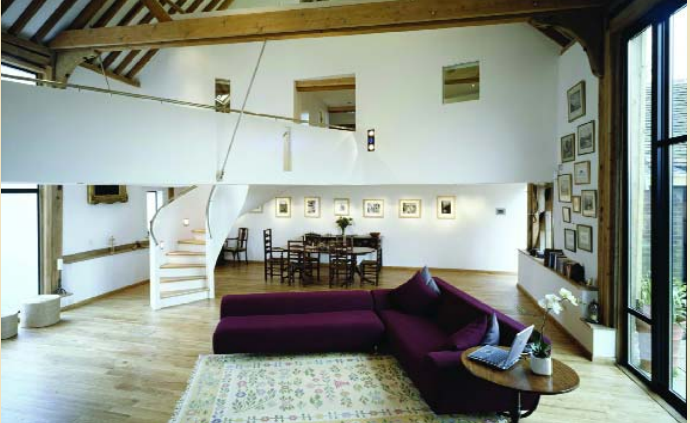
smartcontrols feature project: underfloor heating control, Threshing Barn, Surrey (shown on Channel 4's 'Grand Designs').
