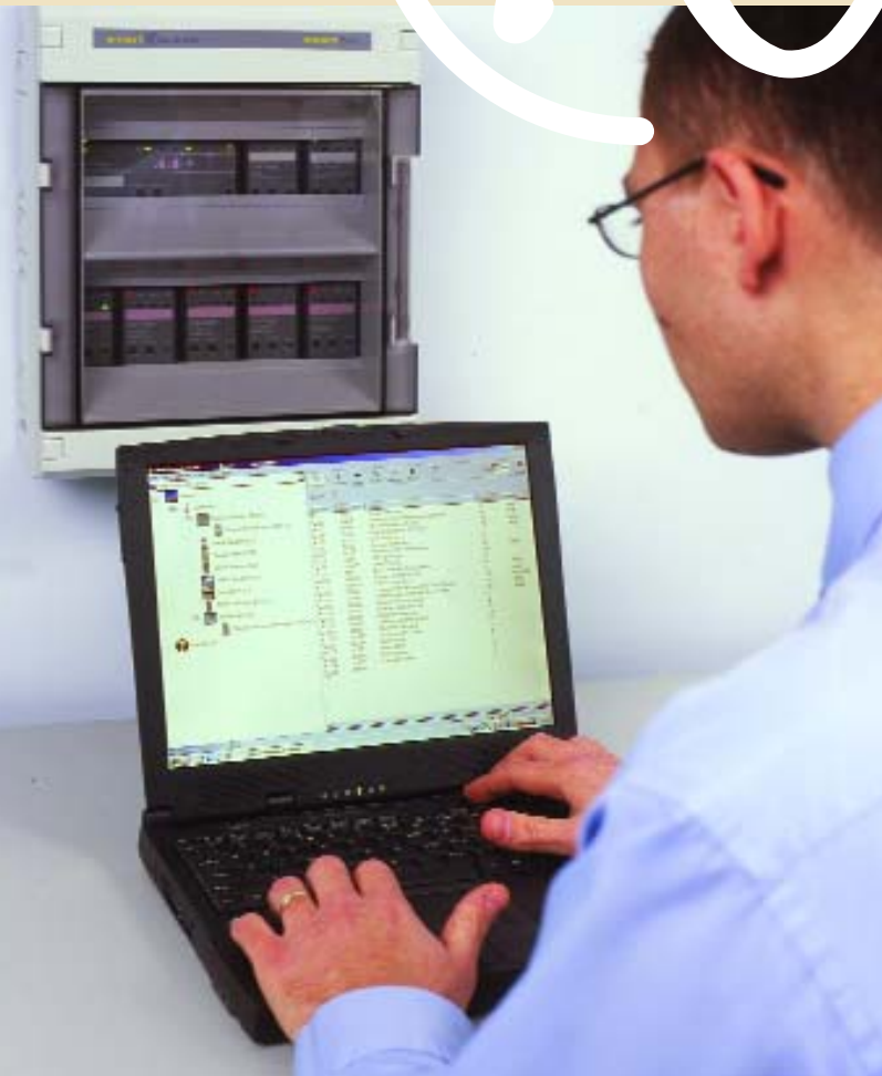
System commissioning in action by a smartkontrols engineer.
