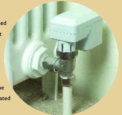
Intelligent actuators eliminate the need for zone valves.
