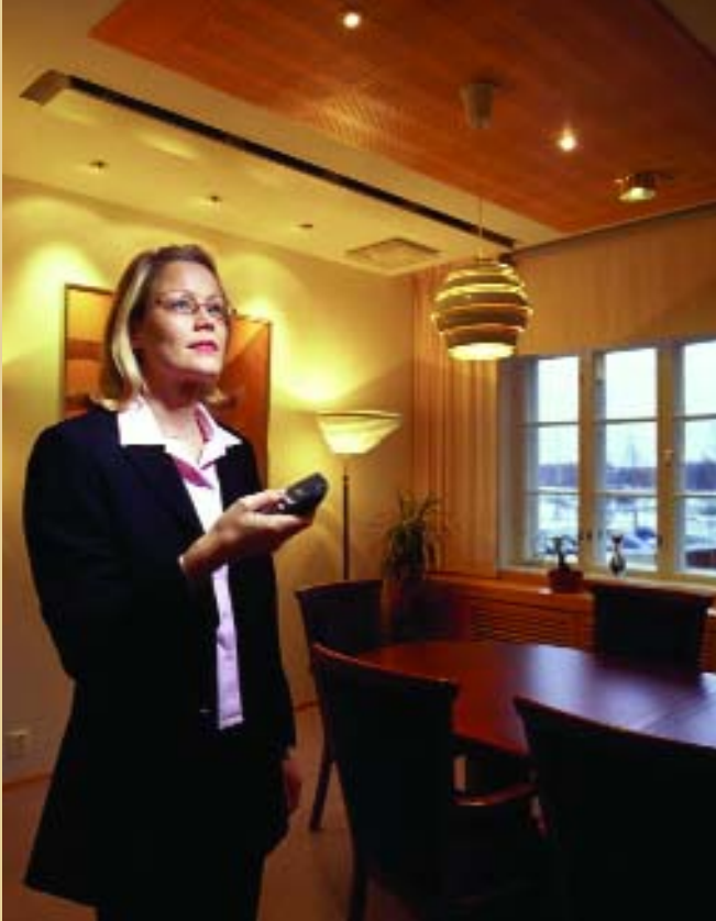
A hand-held transmitter can be used for remote lighting control.
